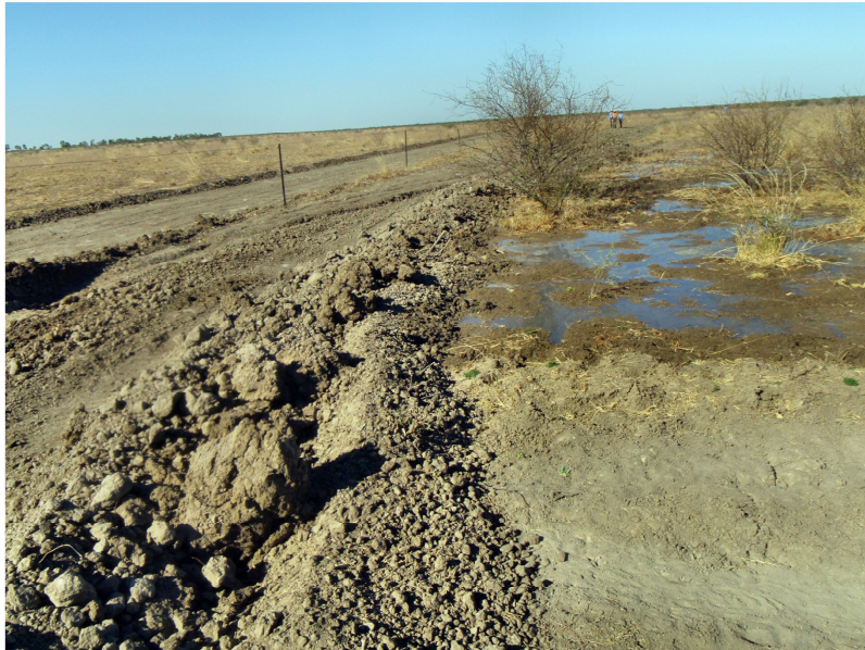
On the ground fence and bunding.
