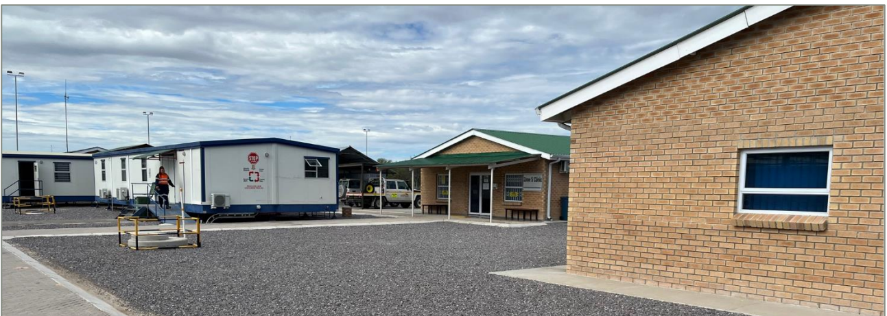
Figure 13-11 Zone 5 medical clinic and emergency service training rooms Source: ERM, 2023
