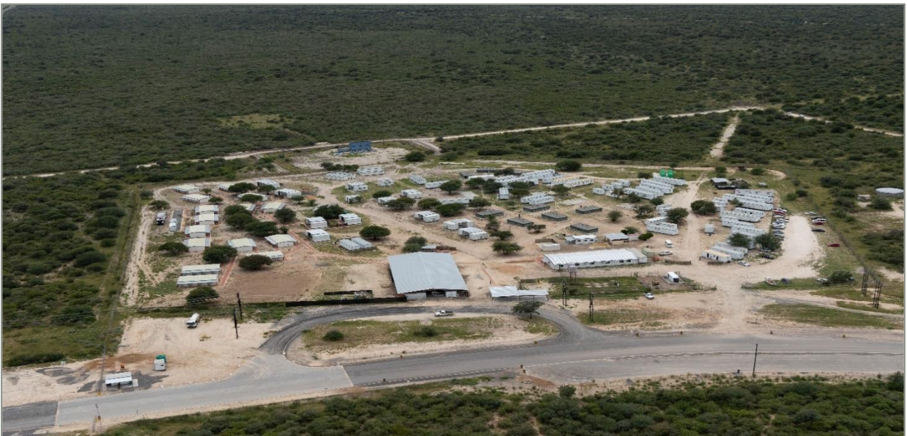
Figure 13-21 Tudika village – Boseto processing plant
