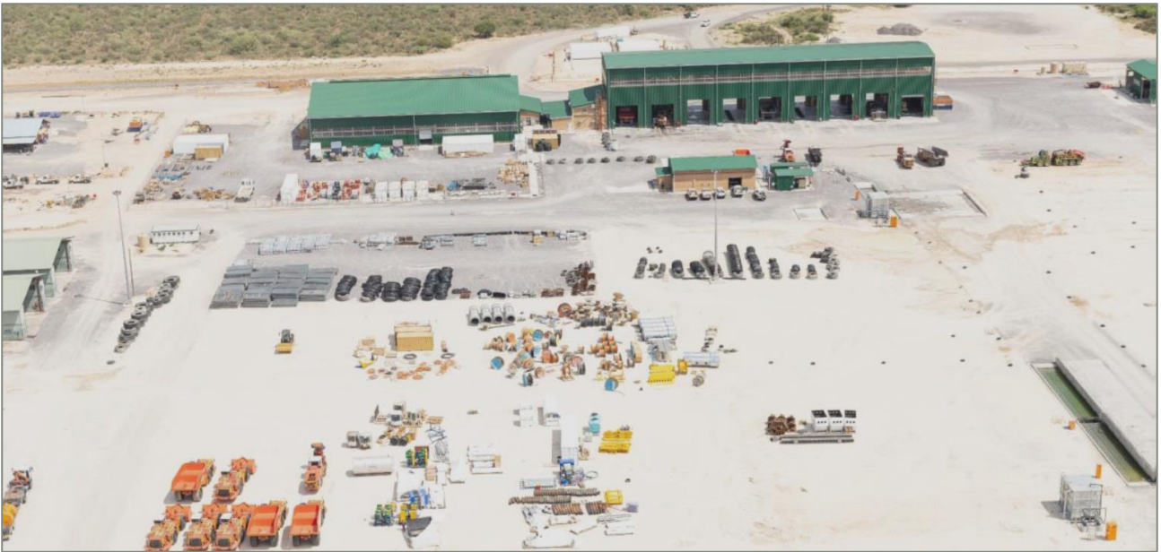
Figure 13-7 HME workshop and associated infrastructure at Zone 5
