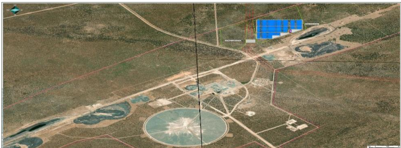
Figure 13-4 Planned solar farm adjacent to the Boseto processing plant
