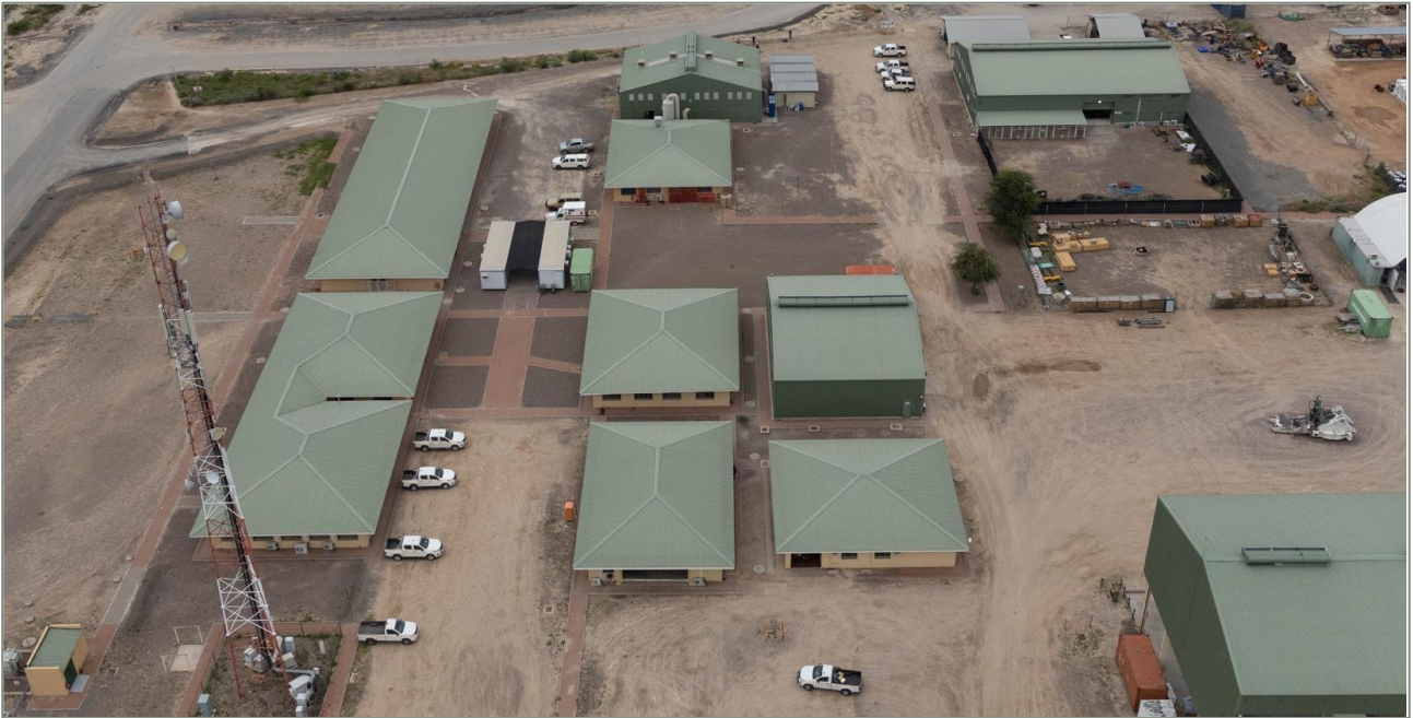
Figure 13-22 Cellular phone and radio communications tower
