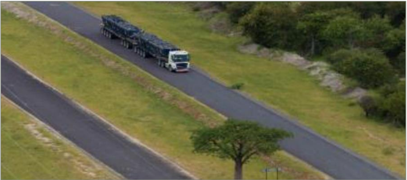
Figure 13-6 Dedicated haul road and associated light vehicle roadway
