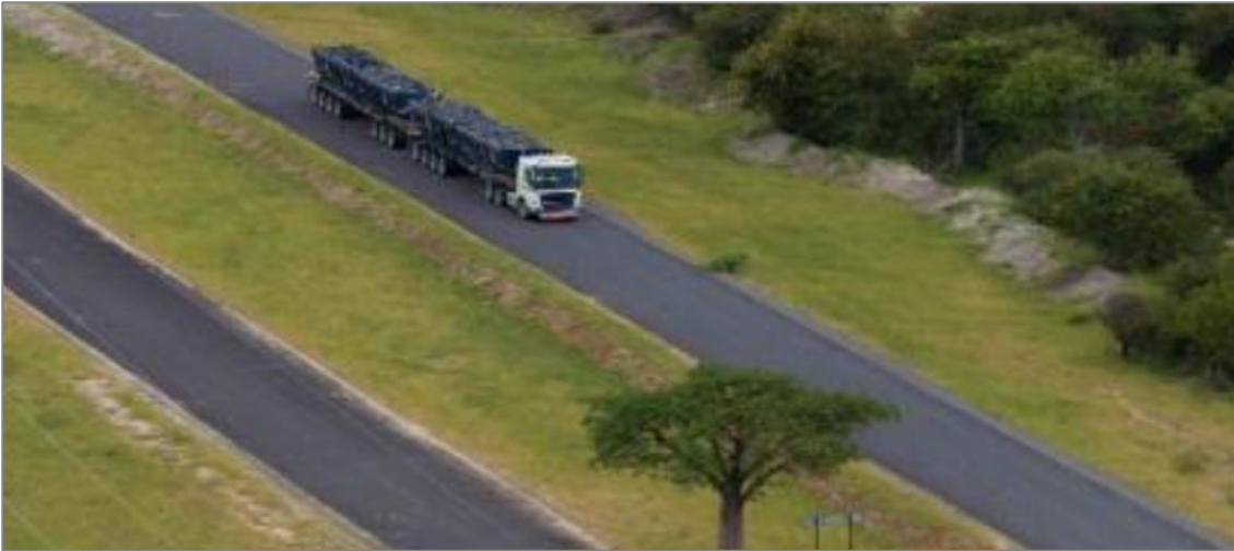
Figure 11-13 Ore haulage road-train on the dedicated Boseto Haul Road
