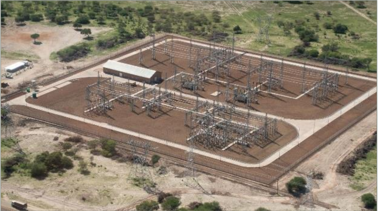
Figure 13-2 Newly constructed site infrastructure
