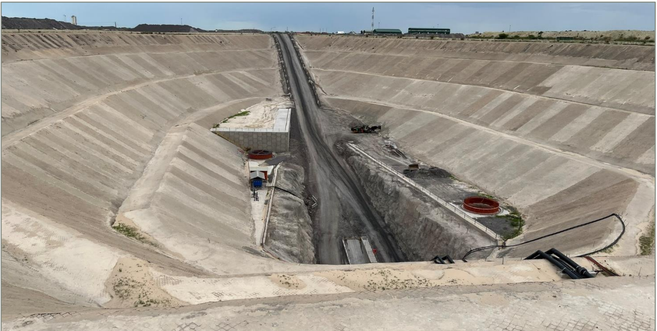
Figure 11-2 Zone 5 boxcut showing mine access and services
