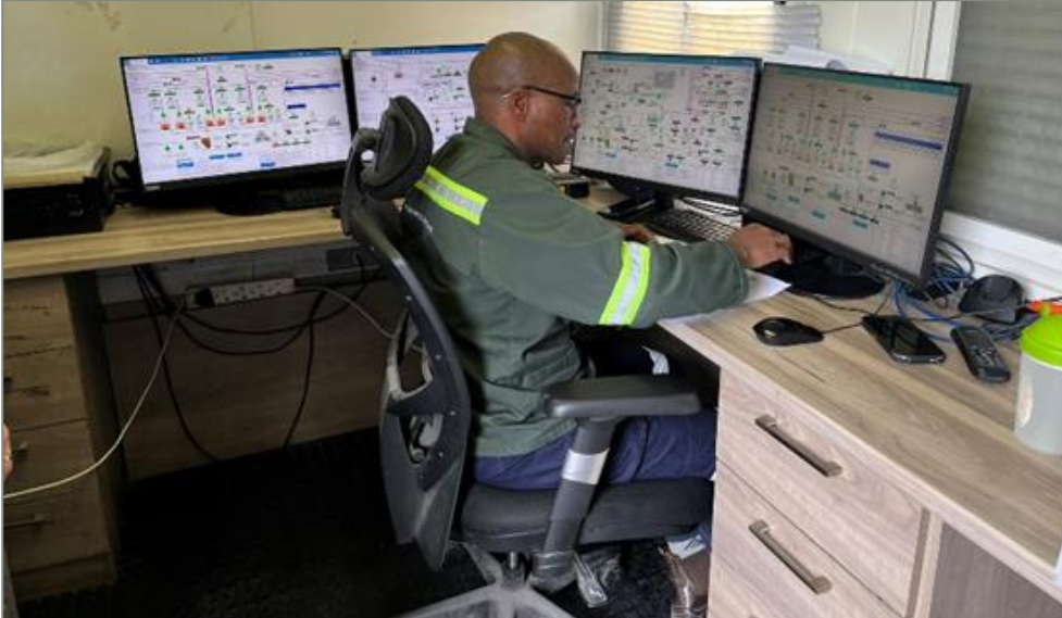
Figure 12-11 Process control room Source: KCM, 2023
