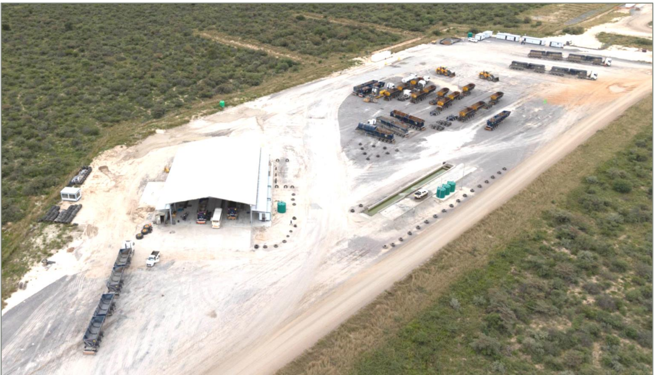
Figure 13-8 Ore haulage workshop and yard (Zone 5)
